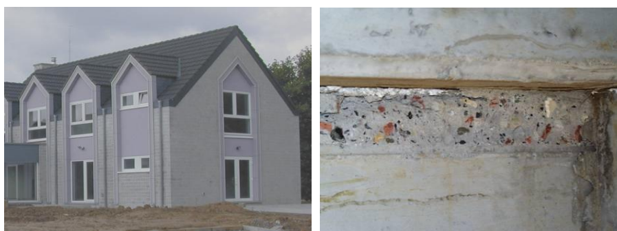
Fig. 2. RecyHouse: overview (l.) & section of a concrete beam, containing recycled C&D waste (r.)
