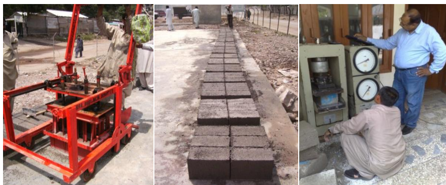
Fig. 6. Concrete block machine & concrete blocks produced & quality control
