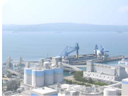
Photograph 1. Overview of centrifugal machine with fly ash silo in Nanao-Ohta coal burning power plant in Ishikawa Prefecture
