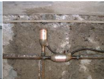
Figure 5 Strain gauges in the reinforcement steel
