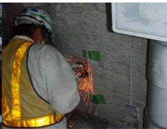
Figure 4 Cutting of reinforcement steel with a grinder
