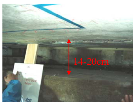
Photo 2. Clearance under hollow slab on abutment
