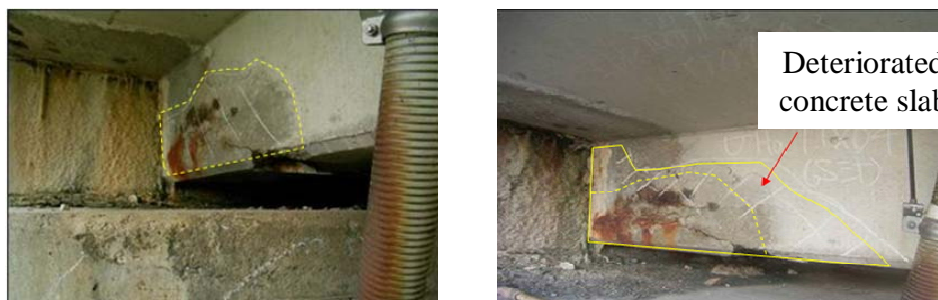
(a) Inspection in 2006
