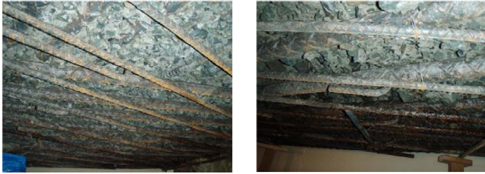
Photo 8. Slab and rebar after chipping deteriorated concrete by water jet
