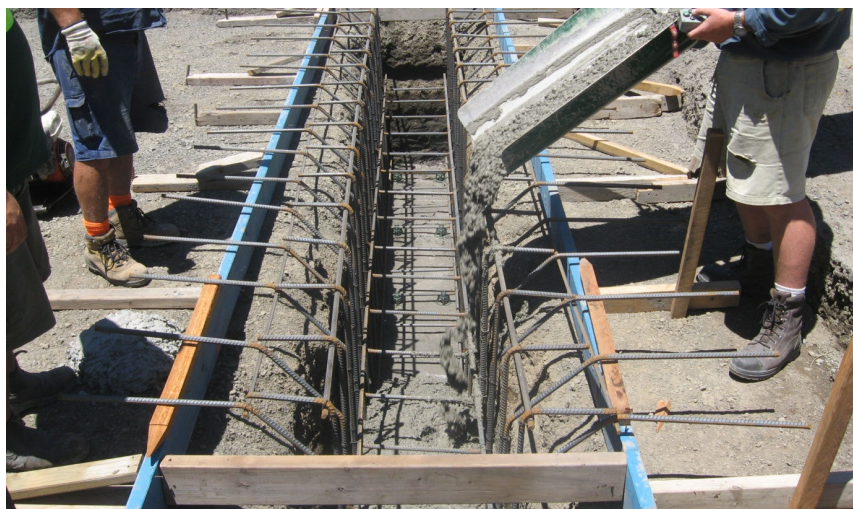
Figure 5. Anchor trench steel / formwork for field trials
