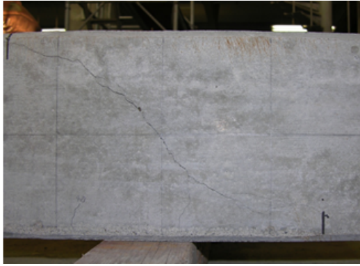
Photo 2. Diagonal tension crack (No.1)
