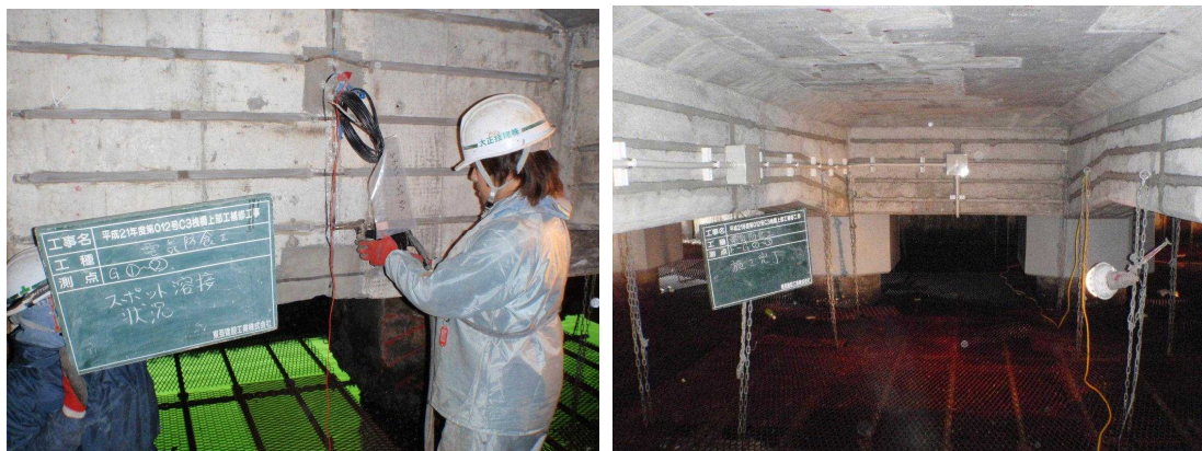
(a) State of spot welding in setting anodes
