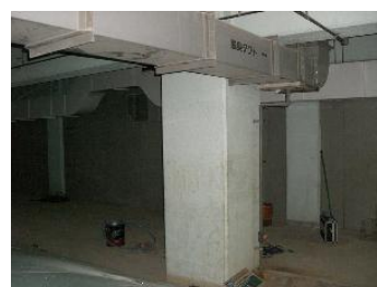
(Pillar of sewage structure)
