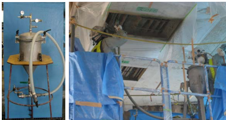
Figure 7. Small spray machine for partial patch repair
