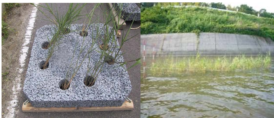
Photo 1 Soaked vegetation base near the steep revetment
