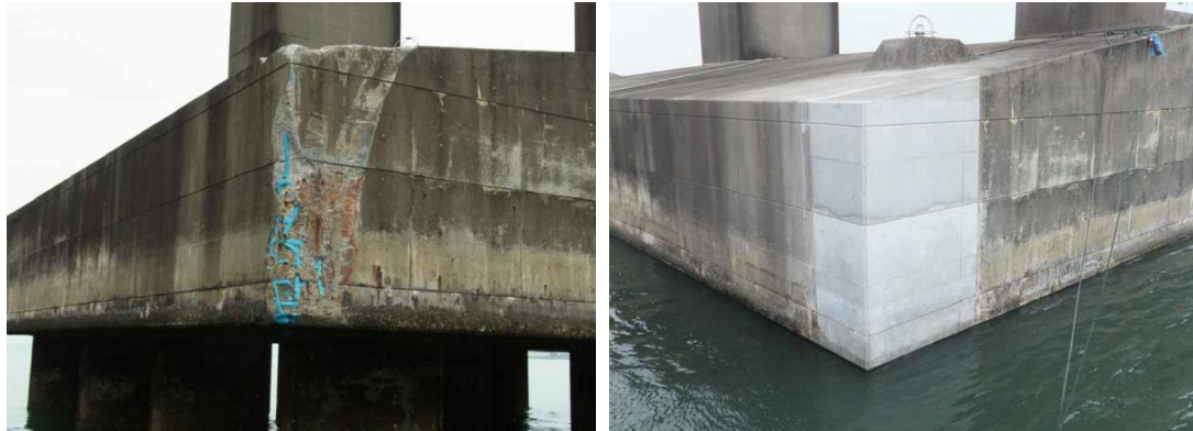
Figure 7 Before (left) and after (right) the repair work of a bridge using pre-packed grout
