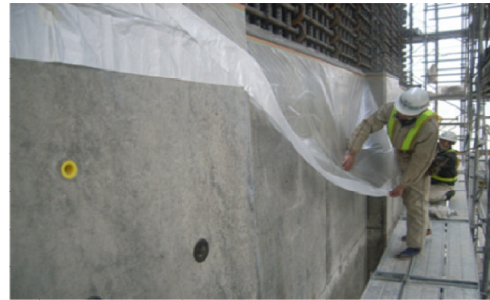
Figure 7. Construction site of pier
