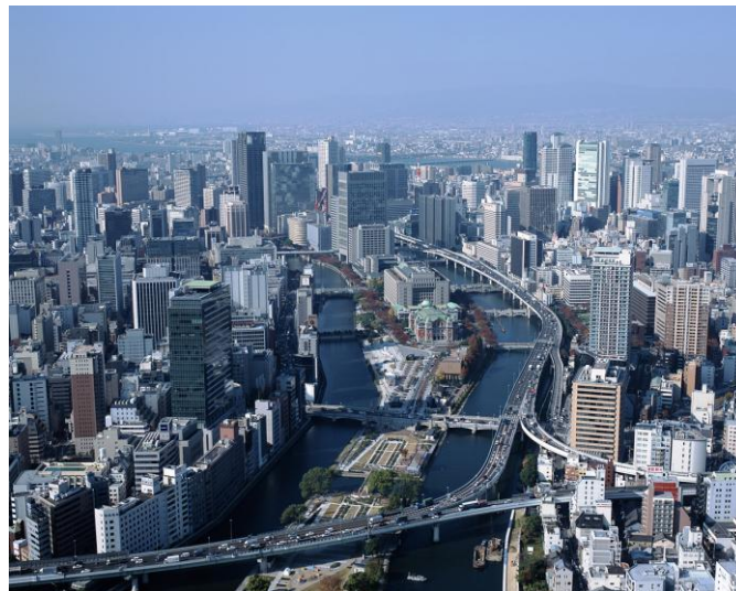
Figure 1. Hanshin Expressway in Central Business District
