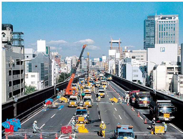
Figure 7. Full Lane Closure Maintenance Works
