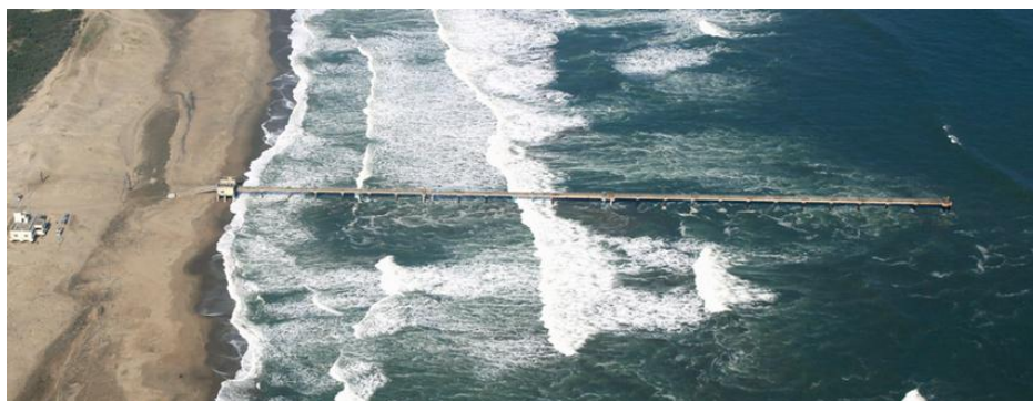
Figure 3. Bird-eye view of the HASAKI pier
