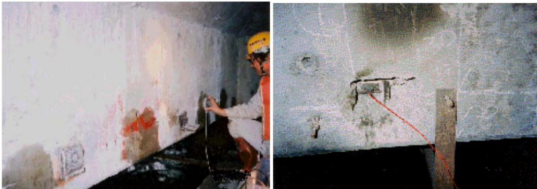
(a) Before installation
