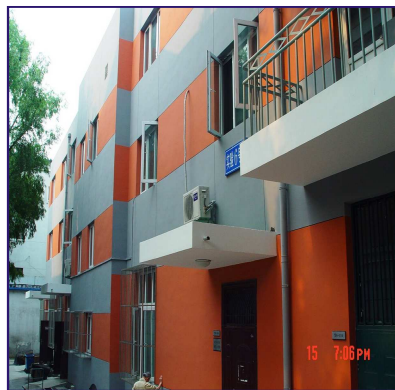
Fig.9. A three-story building constructed with RAC in Beijing
