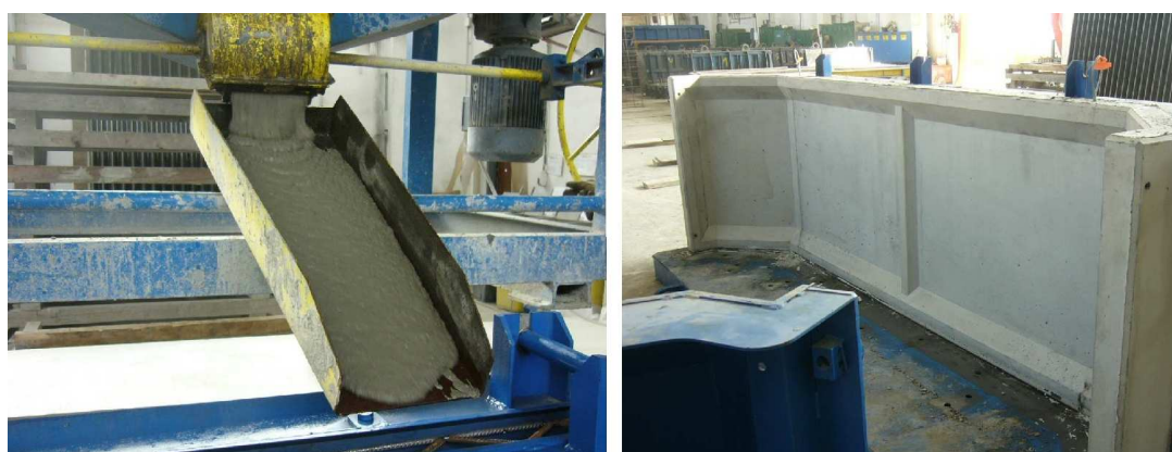
Figure 7. Production of balcony railings from HPFRSSC with ternary binders
