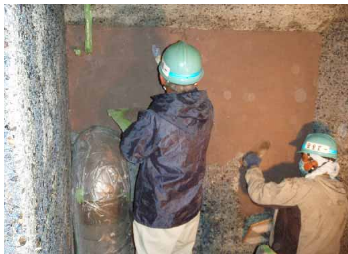
Photo 1. The sulfuric acid-proof mortar construction situation
