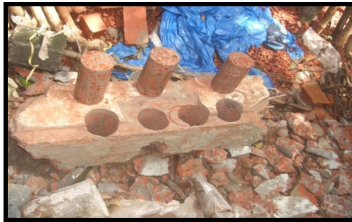
Figure 24. Coring concrete cylinders from demolished buildings
