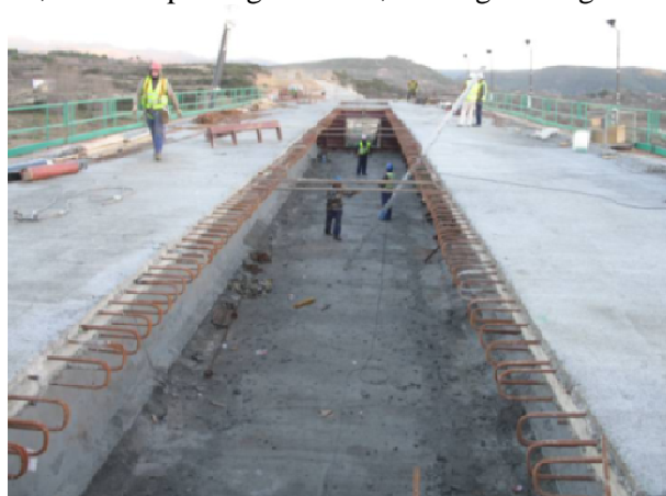
Figure 3. Detail of loop joint connection between phases.
