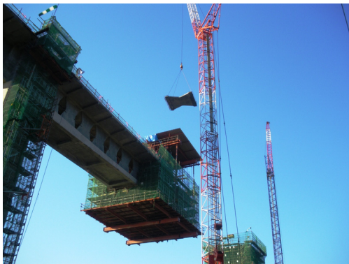
Photo 6. Installation of panels
