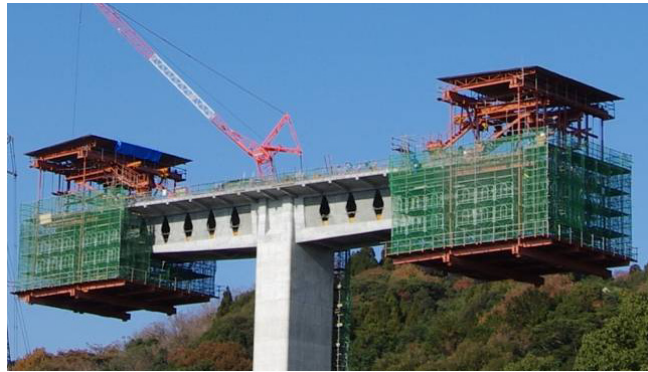
Photo 5. Cantilever construction
