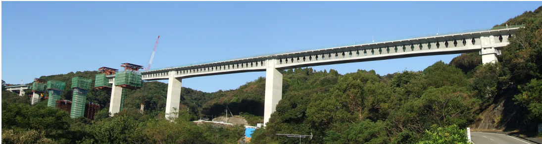
Photo 10. The present construction condition
