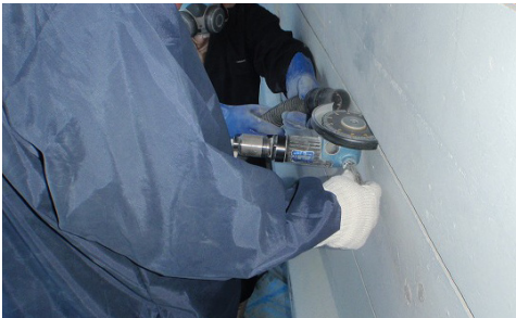
Photo3. Cutting of grooves
