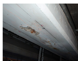
Photo 2. The degradation situation of concrete
