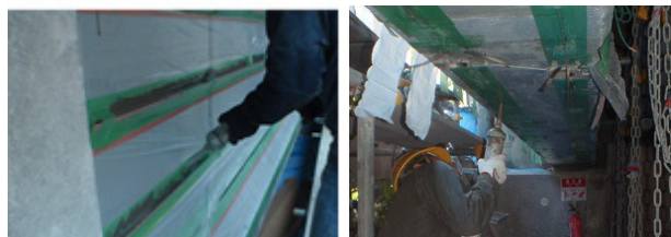
(a) side of the girder (b) Bottom of the girder
