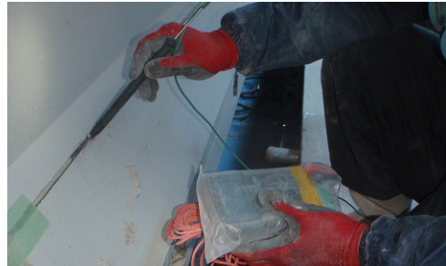
Photo4. In-groove metal detection
