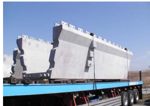
Photo 7 UFC precast block (no rebar inside)
