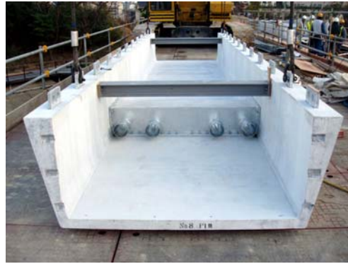
Photo 5 U-shaped girder and PBL
