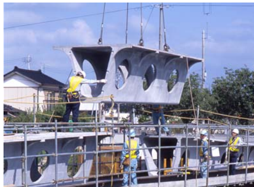
Photo 3 Erection of precast block
