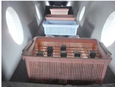
Photo 8 Exposed specimens inside girder
