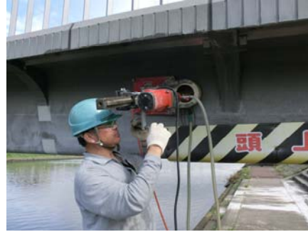
Photo 10 Core drilling in web
