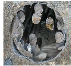
Figure 6. Condition of filling level 4 in E bridge
