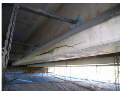
a) Before chipping (G3 girder of the first span)
