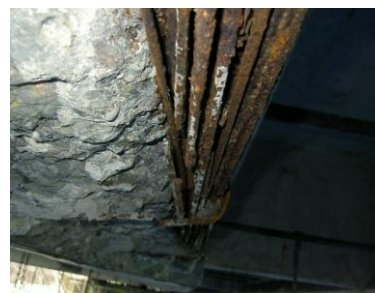
b) After chipping of the same place shown left (breakage of C3 cable)
