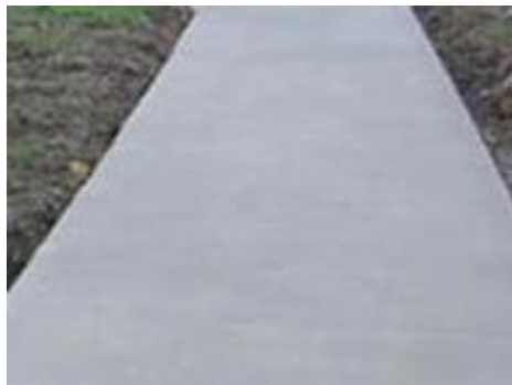
Figure 4: A finished surface of a GPC road ( www.engineering.civil.com )
