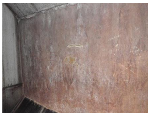
Photo 2. Repaired parts in eight years after the construction
