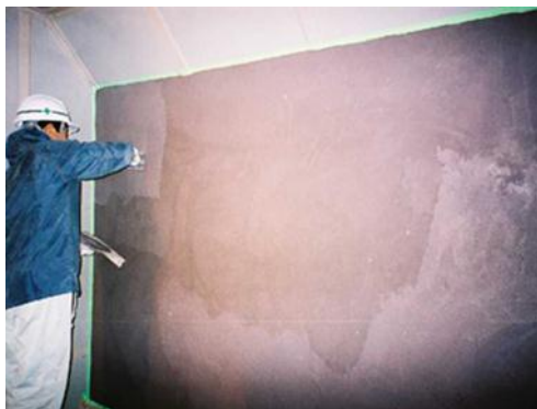
Photo 1. Application of sulfuric-acid-resistant mortar
