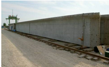
Photo. 6. Real PC road bridge girder
