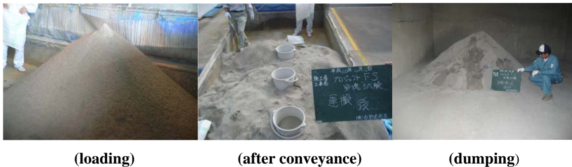
Photograph 1. Loading, conveyance and dumping of FA sand
