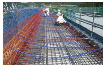
Photo 5. Construction of cast in place slab
