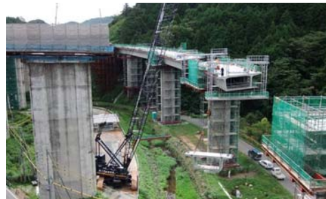
Photo 7. Erection using crawler crane
