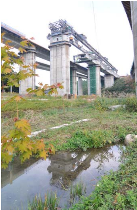
Photo 14. Erection girder and biotope
