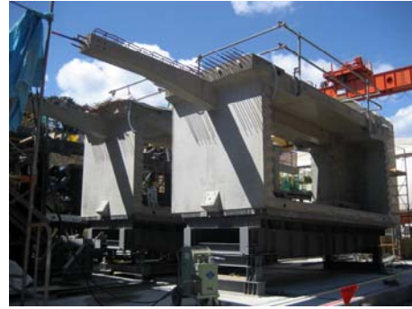
Photo 9. Short-line-match-cast method
