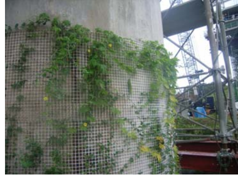
Photo 18. Plantings under the piers
