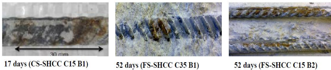
Figure 7. Corrosion inspection in SHCC by destruction at different days
