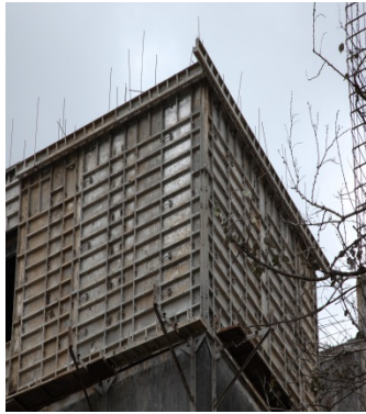
Photo 9 – Modular Formwork
