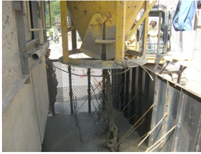
Photo 6 – Placing SDC by kibble
