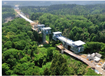
Photo 4 — Placing (cover shot)
