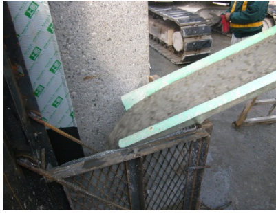
Photo 7 – Placing by chute
