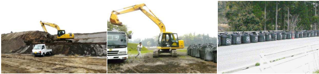
Figure 3. Disposal site carrying accumulated VA (left), work of cramming VA into 1 m 3 -plastick bags (middle), and fixing the bags on sites to prevent VA-debris-flood (right)
