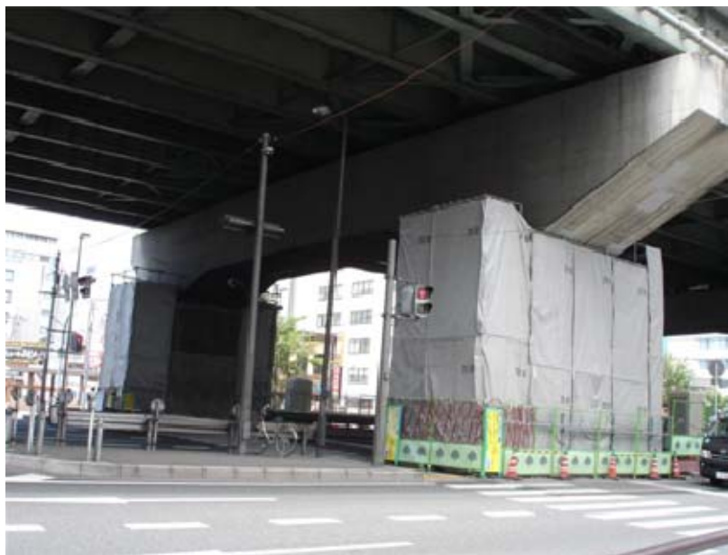
Figure 1. The reinforced concrete rigid frame with two columns (P369)
