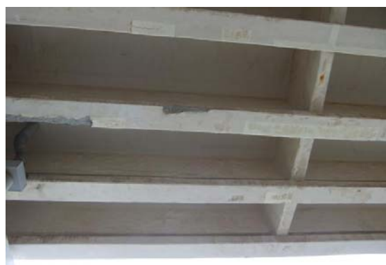
(a) Patching and painting work (7th span)
