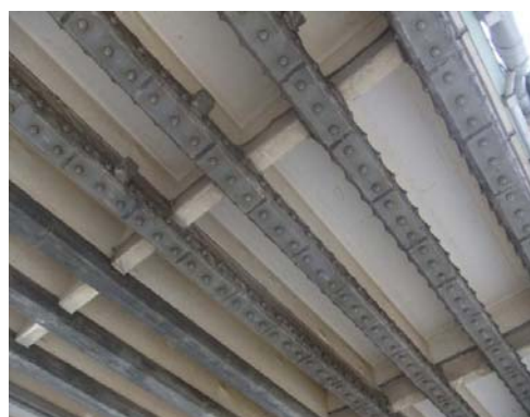
(b) Cathodic protection (8th span)
