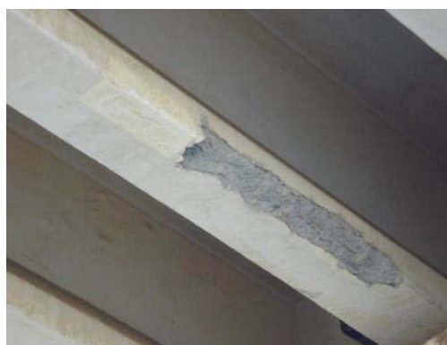
(a) Bridge C (7 years after last repair)
