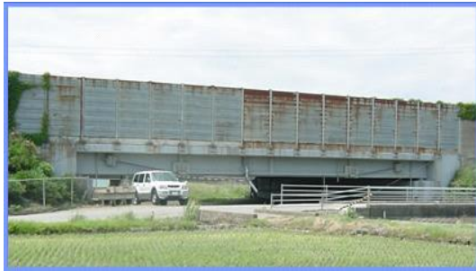
Figure 11. Complete view of monitored bridge at Hokuriku
