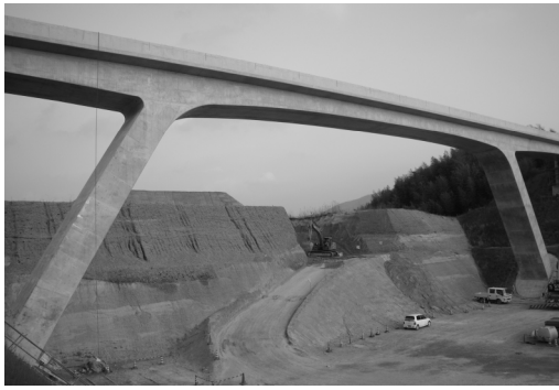
Photo 3. PC strutted rigid frame bridge
