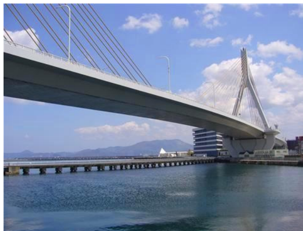
Figure 8. Sea bridge at Tohoku district
