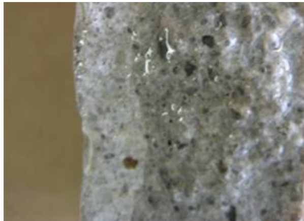
Figure 5. Cross section appearance after coated the surface impregnator (Wet condition)
