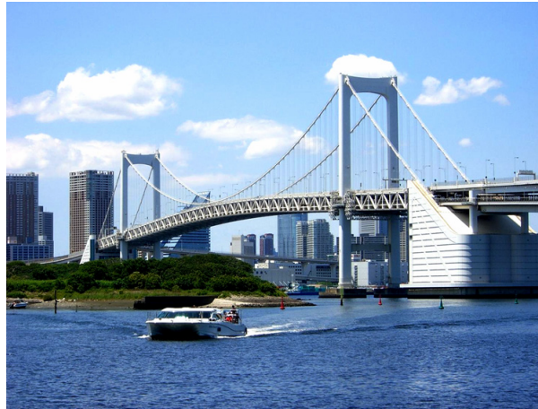
Figure 7. Sea bridge at Tokyo
