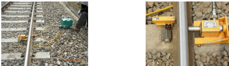
Figure 8. Lateral Resistance Test
