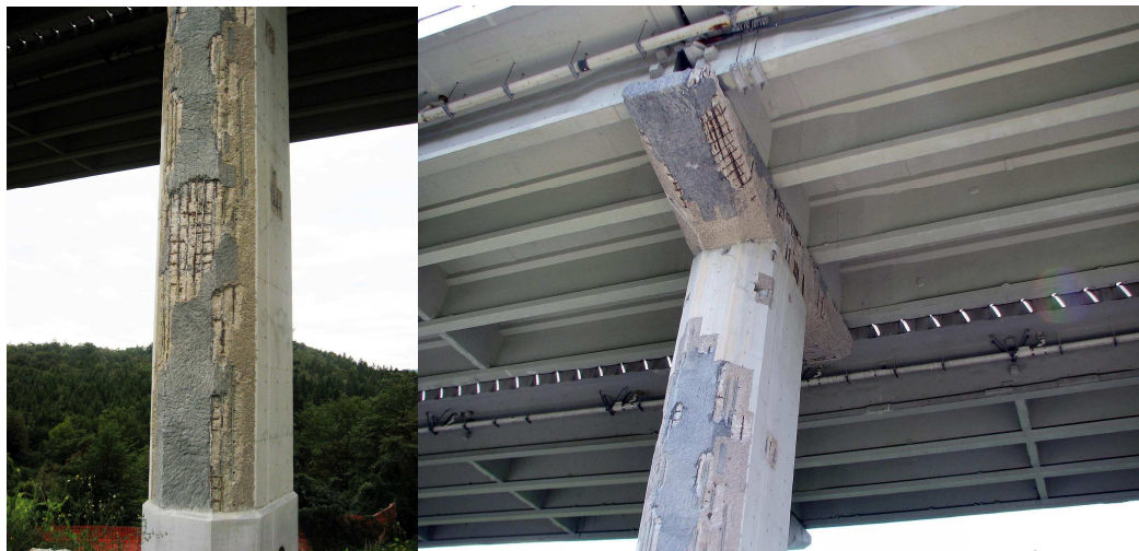
Figure 5: Tall columns and hammerhead crossbeams during the repair work
