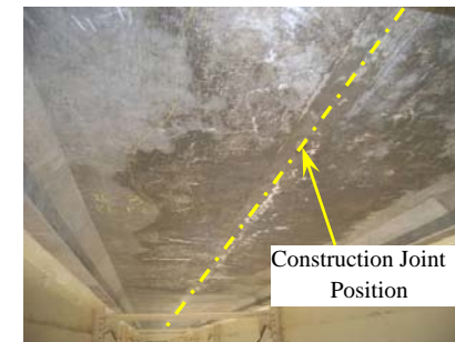
Figure 12. Lower slab surface (Under the ditch of the pavement) Figure 13. Lower slab surface (Under the ditch of the pavement)
