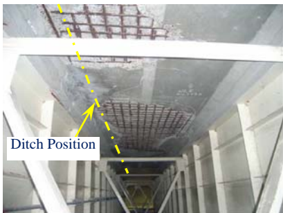
Figure 12. Lower slab surface (Under the ditch of the pavement) Figure 13. Lower slab surface (Under the ditch of the pavement)
