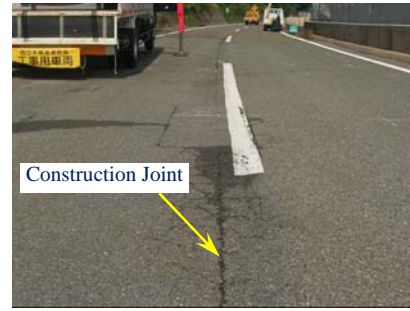
Figure 8. Pavement surface (Ditch) Figure 9. Pavement surface (Construction Joint)
