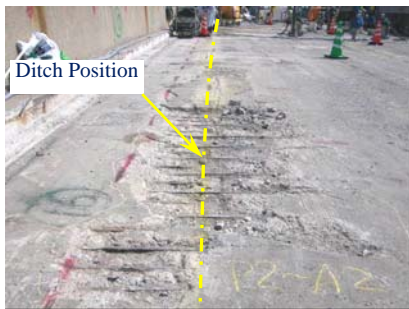
Figure 10. Upper slab surface (Under the ditch of the pavement) Figure 11. Upper slab surface (Under the construction joint of the pavement)
