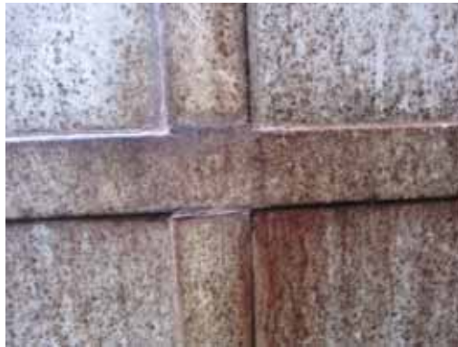
Photograph 7. State of joints with anticorrosive material
