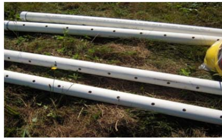
Photo 2: Perforated pipes used to collect infiltrated water
