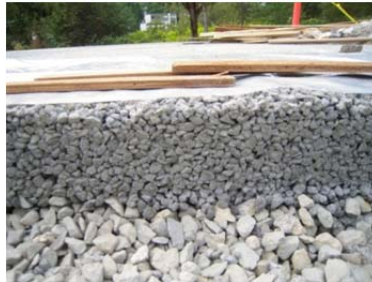
Photo 10: Pervious concrete cross-section after saw cut
