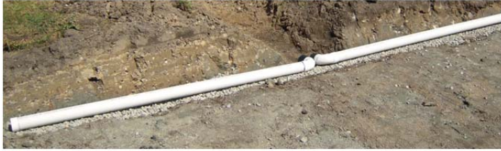
Photo 3: Perforated pipes above the subgrade
