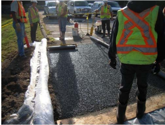
Photo 8: The second roller giving the desired finish of the concrete
