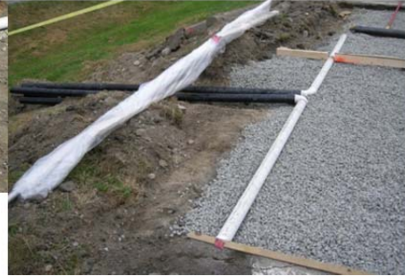
Photo 4: Perforated pipes on top of crush connecting to ABS pipes
