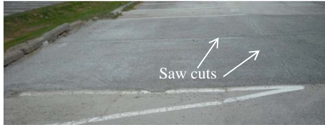
Photo 11: Cured concrete slab with saw cuts
