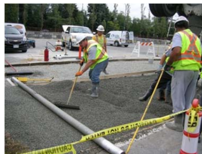
Photo 7: Roller screed and leveling
