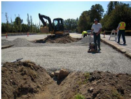
Photo 5: Compaction of clear crush and simultaneous excavation
