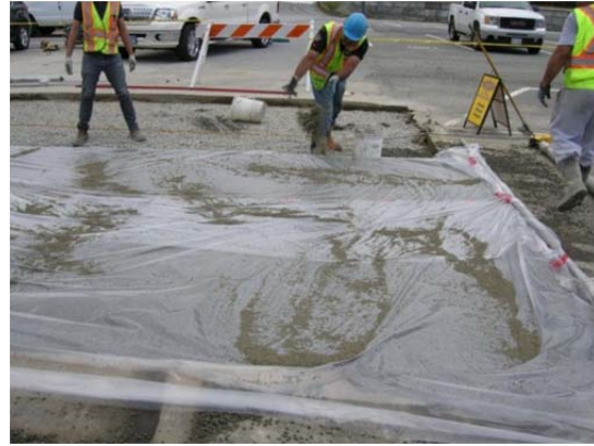
Photo 9: Finished concrete slab (Bay 1) covered with polyethylene sheet
