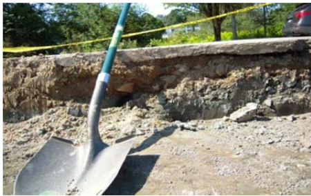
Photo 1: Pavement cross-section observed during excavation
