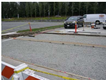
Photo 6: Site with formwork and compacted crush
