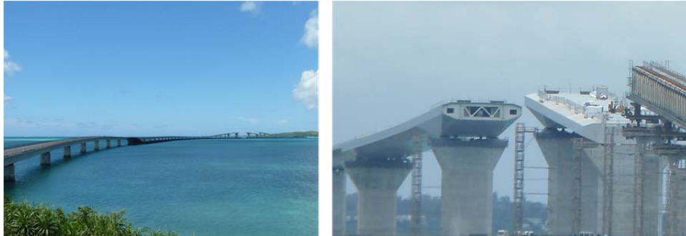
Fig.5 The IRABU GREAT bridge under construction. Courtesy by Prof. Tomiyama
