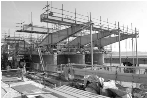
Photo 1. Construction of box girder
