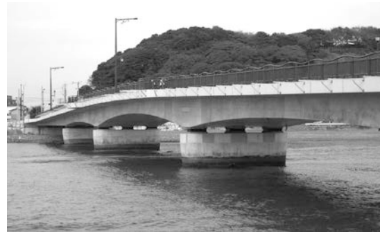
Photo 2. Side view of the bridge
