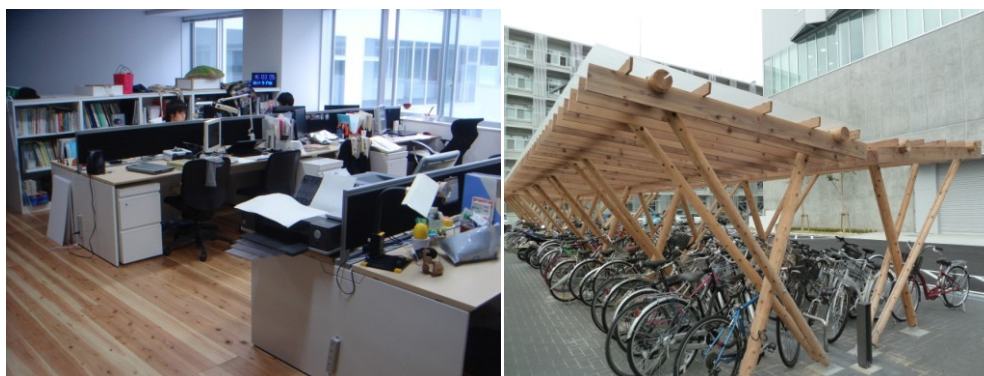
Figure 8. Wood utilization on Nagoya University campus (Cedar flooring and bicycle parking)
