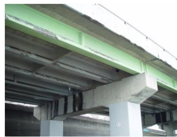
Photo 6. Degradation due to the use of insufficiently desalinated sea sand,
