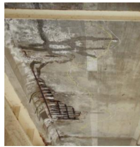
Photo 5. Chloride induced deterioration (de-icing salt)
