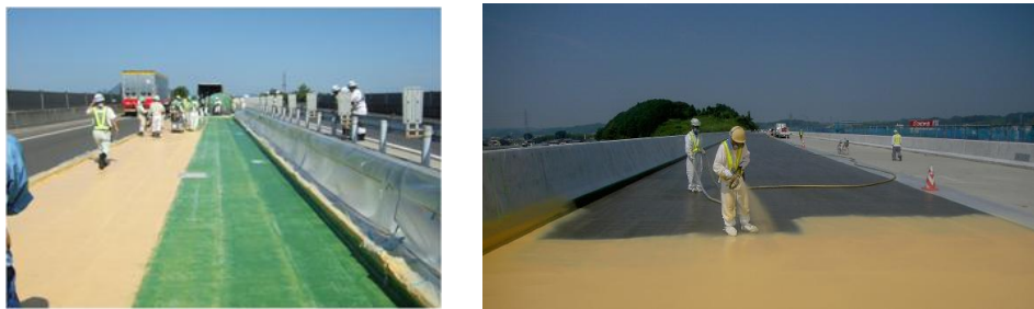
Photo 15. Laying waterproofing
