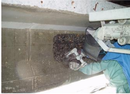
Photo 11. Chipping with the water-jet
