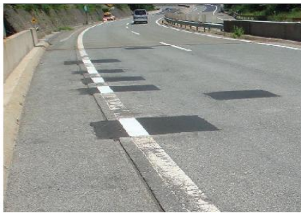
Photo 5. Chloride induced deterioration (de-icing salt)
