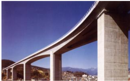
Photo 1. Principal PC Bridge (OKAYA Viaduct)
