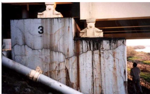
Photo 7. Alkali-aggregate reaction
