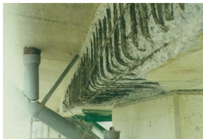
Photo 6. Degradation due to the use of insufficiently desalinated sea sand,
