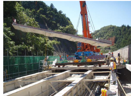
Photo 14. Replacement floor slab
