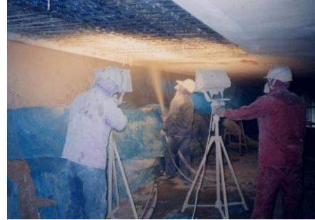
Photo 12. Patching or Increasing thickness by Shotcrete
