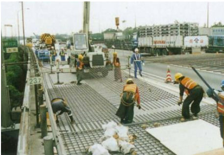
Photo 13. Floor slab overlaying
