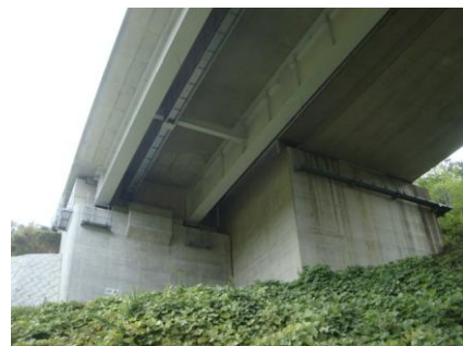
Photo 2. RC Floor Slab/Multiple Main Girder Photo 3. PC Floor Slab/Minimum Main Girder
