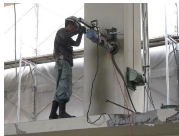
Figure 2. Core Boring(2F)
