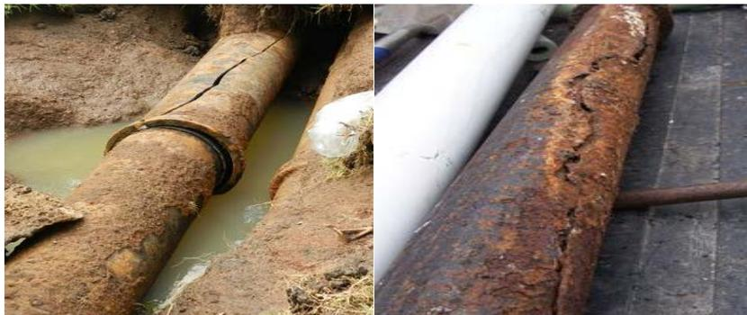
**Figure. 1. Failure due to inclined cracks [From URL]**
