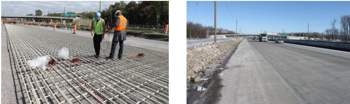
Figure 6. GFRP Bar Placement in Center Lane in Highway 40, Montreal, QC, Canada
