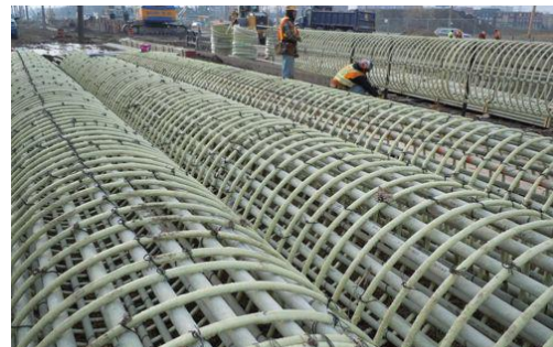
(b) GFRP reinforcing cages for soft-eye
