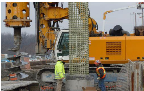
(c) Handling and lifting the GFRP soft-eye
