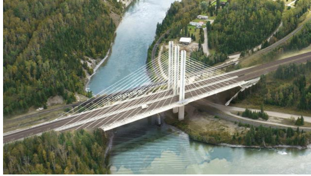
Figure 2. Nipigon Cable-Stayed Bridge, ON, Canada
