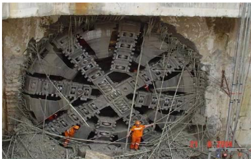
(a) TBM cutting through FRP-RC wall
