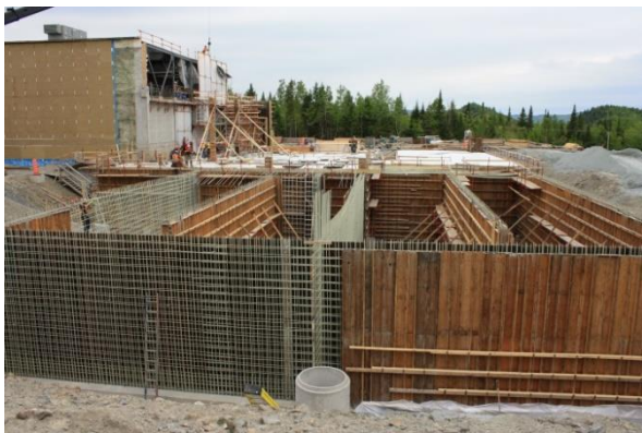
(a) FRP reinforcement of the wall
