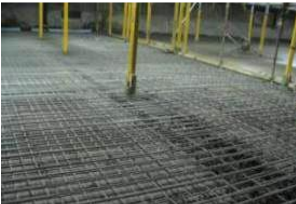
(a) Laurier-Taché parking garage
