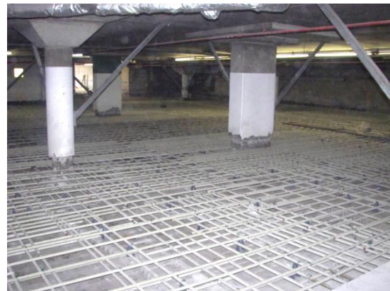
(b) La Chancelière parking garage
