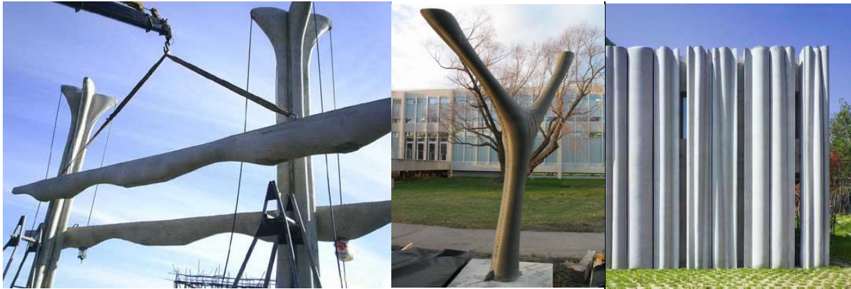
Figure 1. Examples of Fabric-Formed Concrete (Courtesy of Mark West)
